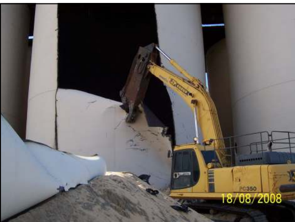
Lower part of tank being sheared by PC350 Excavator with shear.
